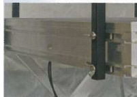
Bridage garde-corps / Handrail fixation
