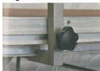
Bridage garde-corps / Handrail fixation
